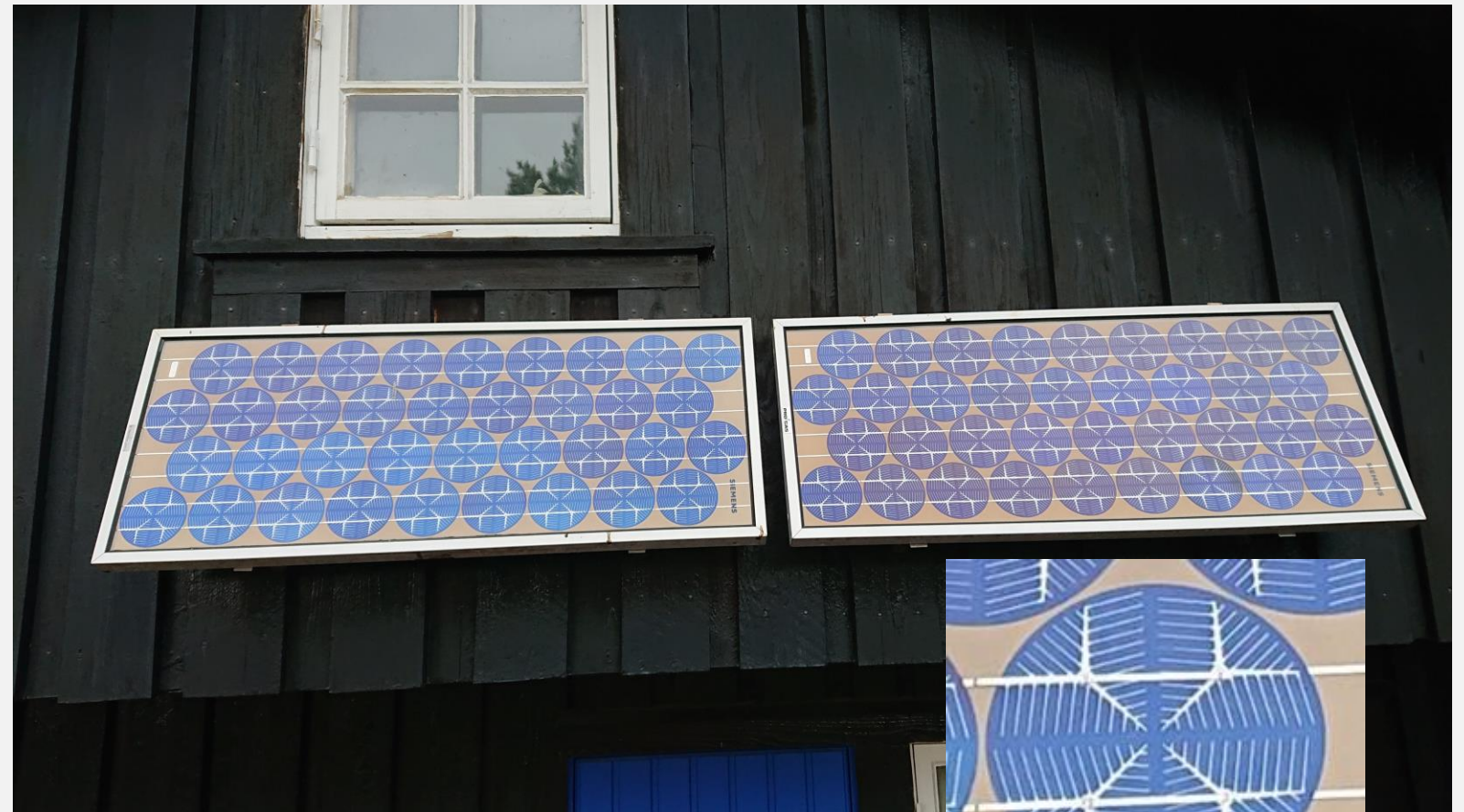
Solar panels from around 1982, still going strong and producing all necessary energy for a cabin in Telemark region, Norway
